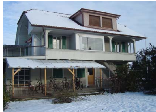
Rychiger house shortly before the pull down in January 2010
